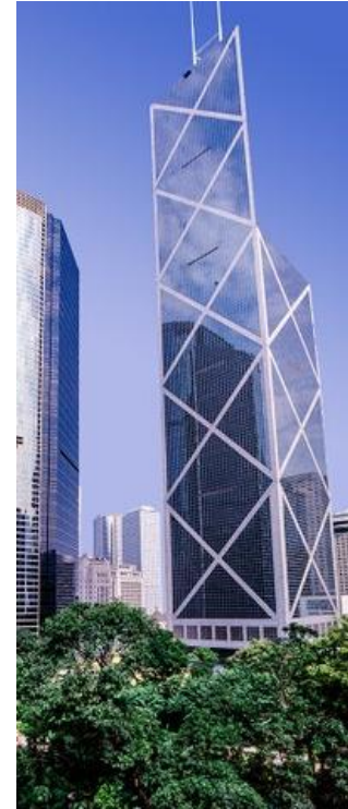
Figure 97 : Bank of China (Hong Kong) Ieoh Ming Pei 1990. Source: © Getty / Photo John Seaton Callahan.
