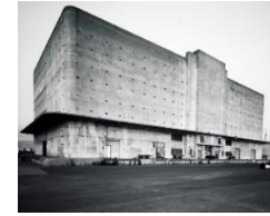
Figure 229 : Effet massif (General Warehouse – Richard Kaiser Naval Shipyard, near San Francisco.)
