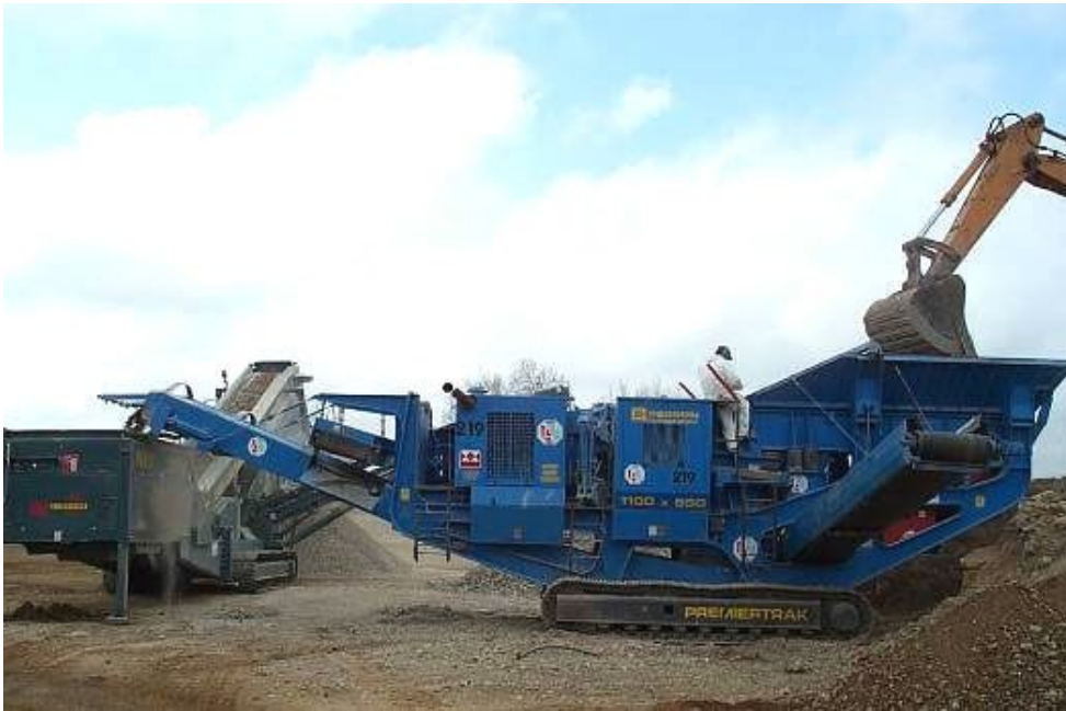
Concassage - Criblage mobile
