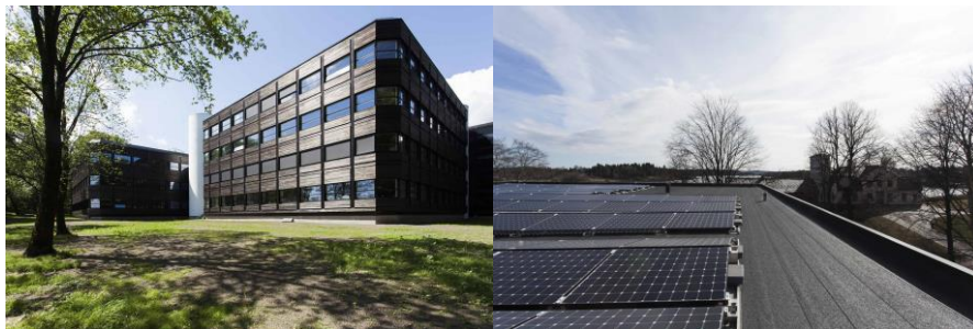
Figure 6 : powerhouse kjoerbo oslo norway 7
